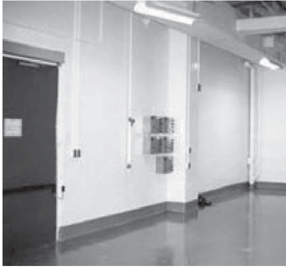
FIGURE 6 A CMU wall treated with block filler and epoxy finish to provide a smooth, cleanable wall surface. (Courtesy of Niagara Walls.)
