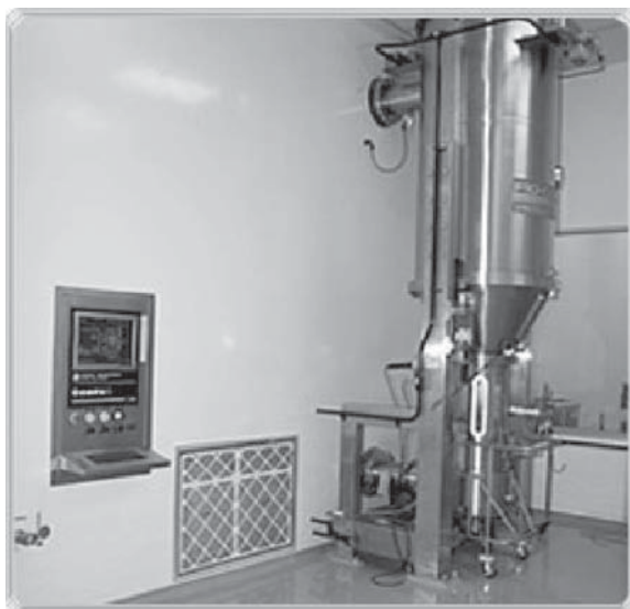
FIGURE 8 A modular wall system has been installed in a manner that provides a smooth surface for cleaning. The fit of the components and the method of sealing are important when a modular wall is selected. (Courtesy of Portafab.)
