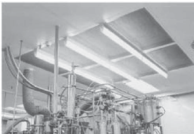
FIGURE 10 An area of HEPA filters is installed above a process machining. Tear drop lighting is used to permit maximum filter coverage. A monolithic ceiling construction of gypsum panels suspended from a framework. The panels are finished with an epoxy coating compatible with cleaning/sterilization procedures. (Courtesy of CleanTek.)
